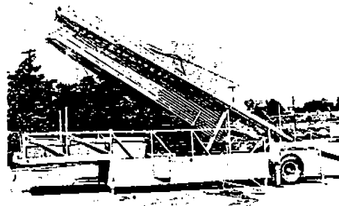
2 Towers Raised to a Convenient Height to Pull Pins and Let Wind Brace Down.
